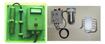
Radioactive Releases Monitoring System was redesigned to meet the requirements of continuous monitoring of releases during normal operation and in accident conditions, ensuring sensibility and all range of measurements for expected radioactive species gamma emitters gases and aerosols. This system was designed and built by a provider licensed by Regulatory Authority on contractual basis.
